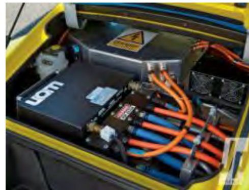
EV Battery Assy
